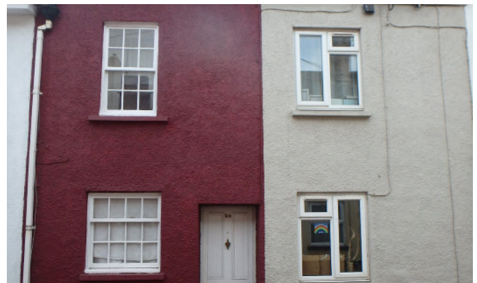
Original and replacement windows side by side
