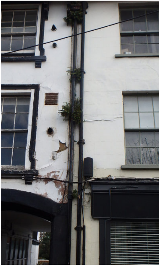
Blocked and overflowing downpipe
